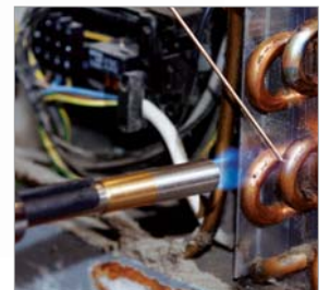
Hard soldering in refrigeration and climate control
