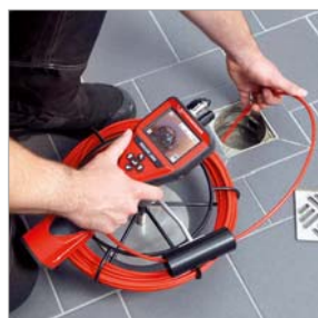
Inspection from floor drains
