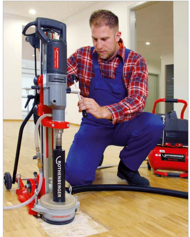
Clean work in enclosed rooms
