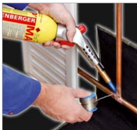
Soft soldering in heating installation
